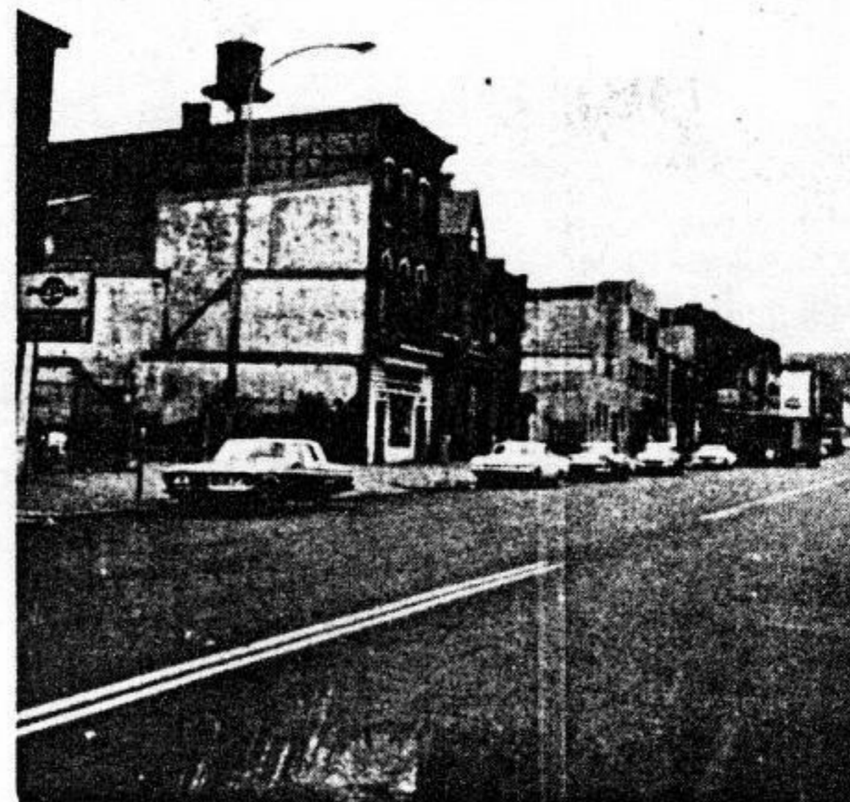
Substandard Buildings 3300 Block, Market Street
