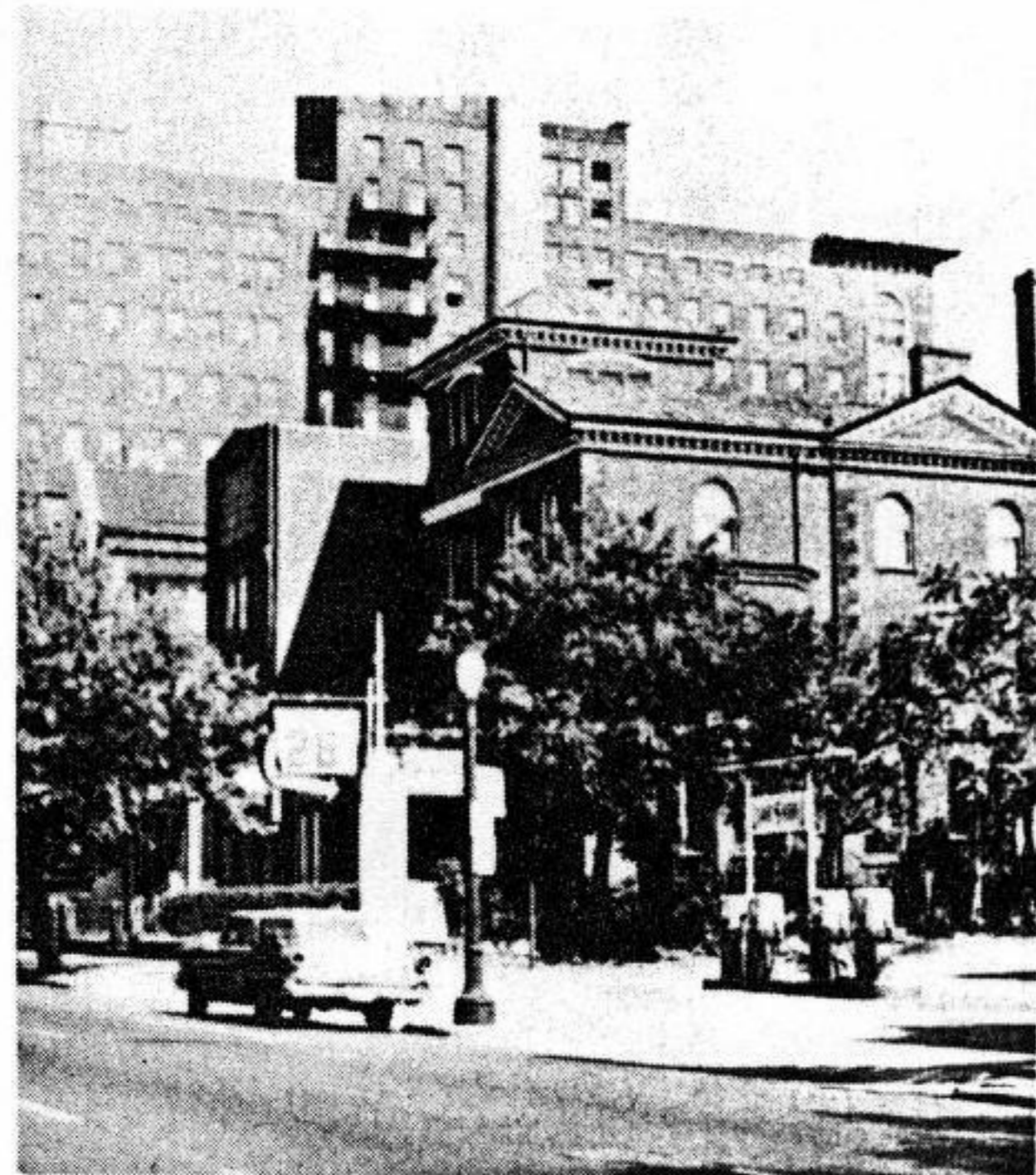
Incompatible land uses, 3900 Block, Chestnut Street
